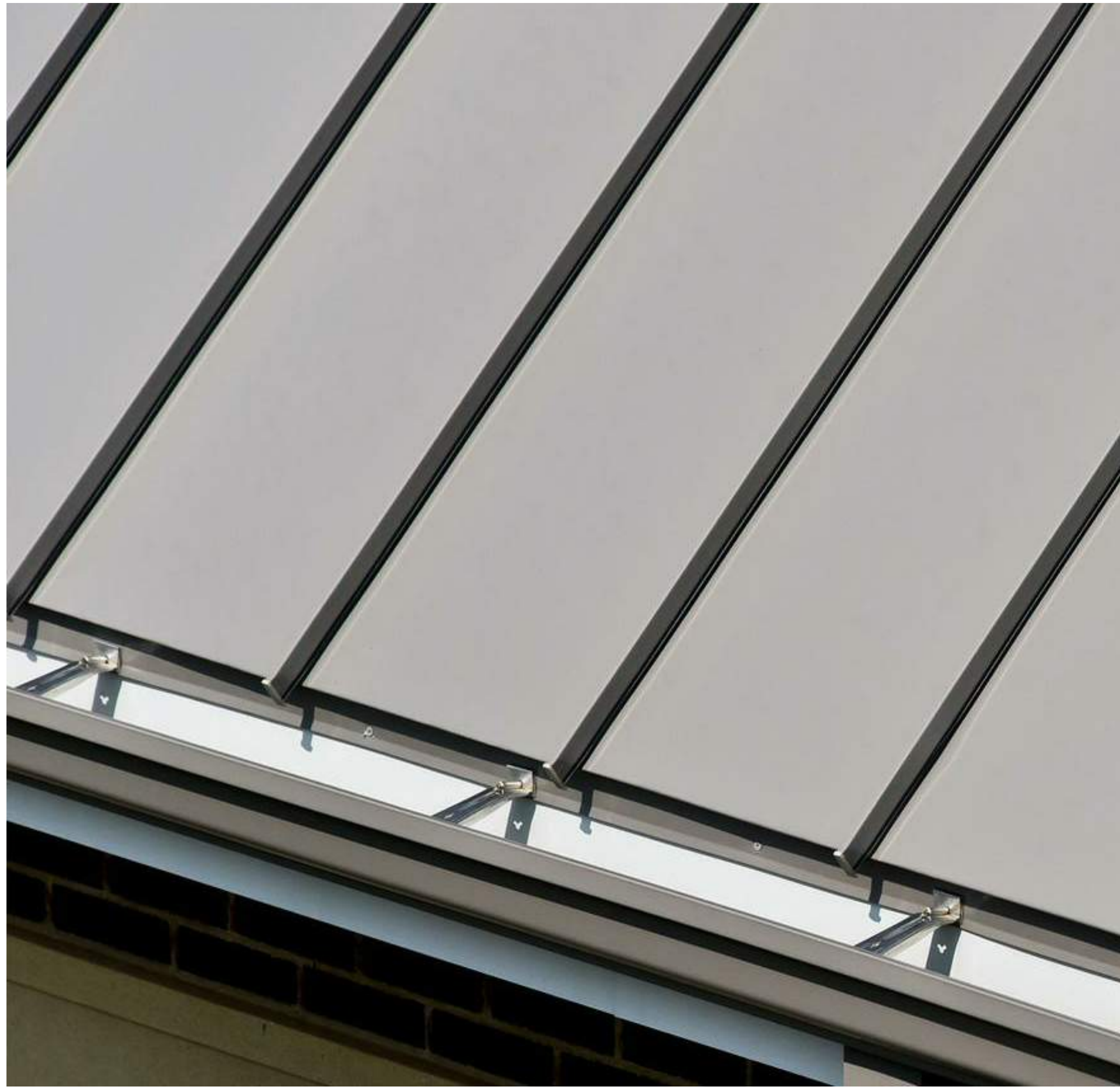
STANDING SEAM METAL ROOFING
